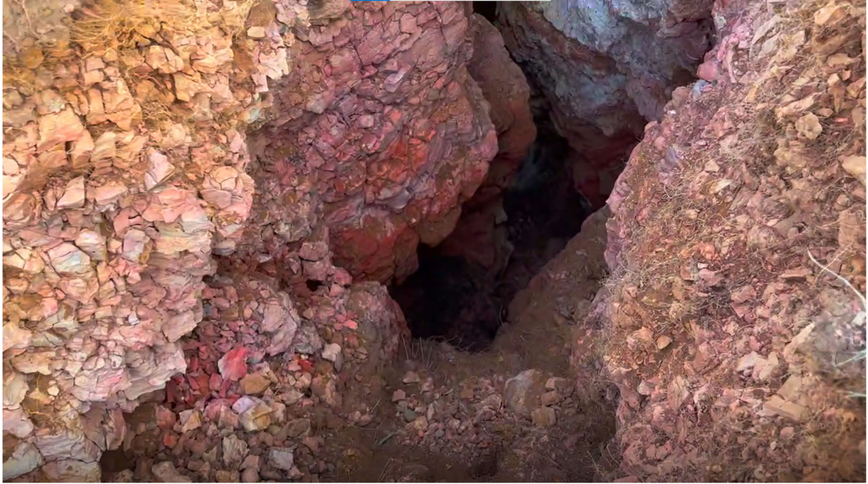
Figure 6. Subsidence crack, 2 Lazy 2 Ranch, Sec. 22, T7N, R27E (November 4, 2022)
