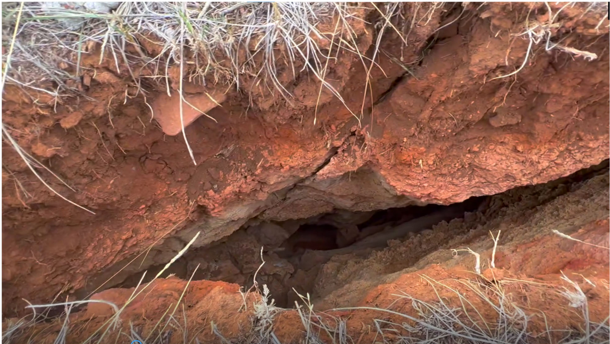
Figure 3. Subsidence cracks, 2 Lazy 2 Ranch, Sec. 22, T7N, R27E (November 4, 2022)
