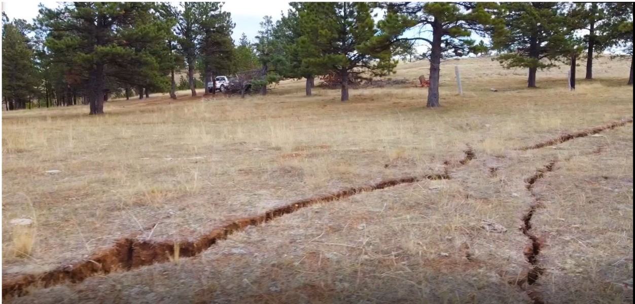
Figure 1. Subsidence cracks, 2 Lazy 2 Ranch, Sec. 22, T7N, R27E (November 4, 2022)
