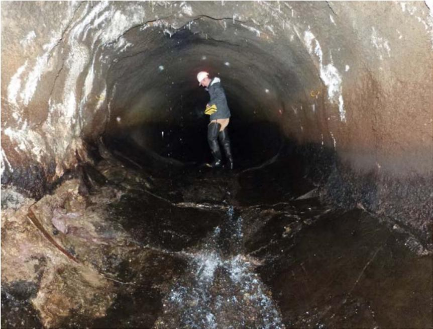
**FIGURE 2.11** Photo of heave in the tunnel. The tunnel diameter was originally 11 feet. The man is standing on the heaved portion of the tunnel. SOURCE: Britton et al., 2016a.
