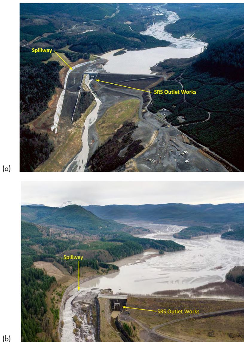
**FIGURE 2.12** The SRS and the sediment plain (a) in approximately 1990 prior to the outlet works reaching their upstream capacity (b) and after reaching capacity. Note that water is now diverted over the spillway in the left of the photo. SOURCE: USACE.
