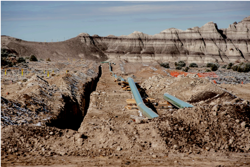
Above, Mancos shale fracking operation. Below, oil pipeline construction associated with Mancos shale development. Photos by Carlan Tapp.
